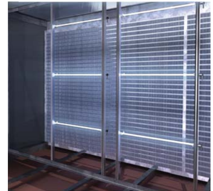
CCX48 3X2 Array System Rack-mounted on Cooling Coil
