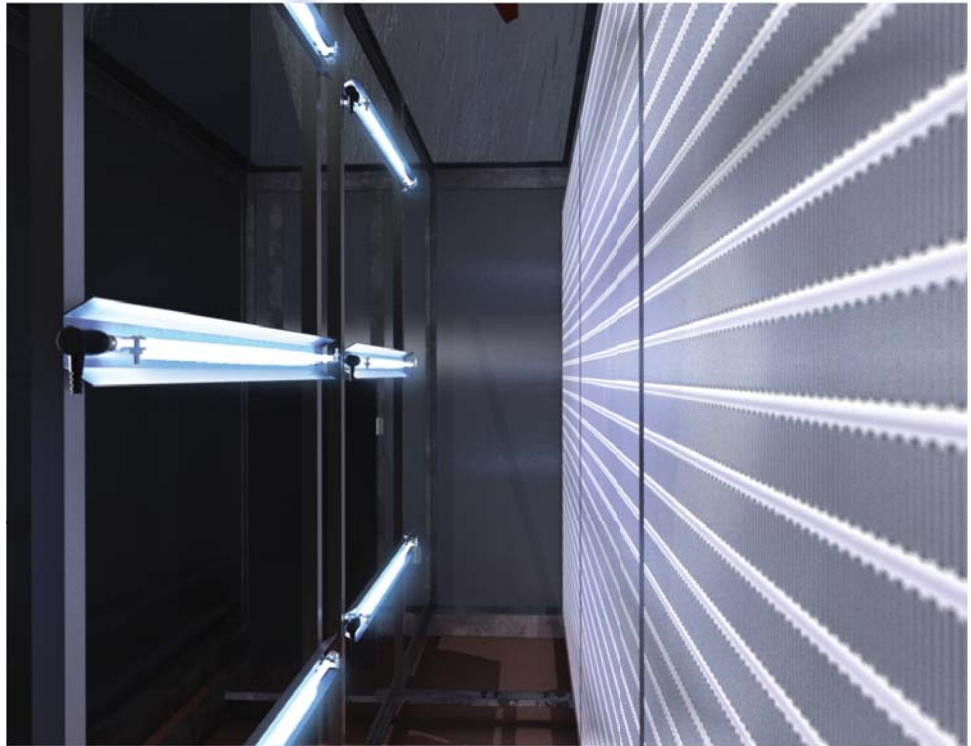
CCX64 3X2 Array System Rack-mounted on Cooling Coil
